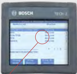
Multiplex network module status
